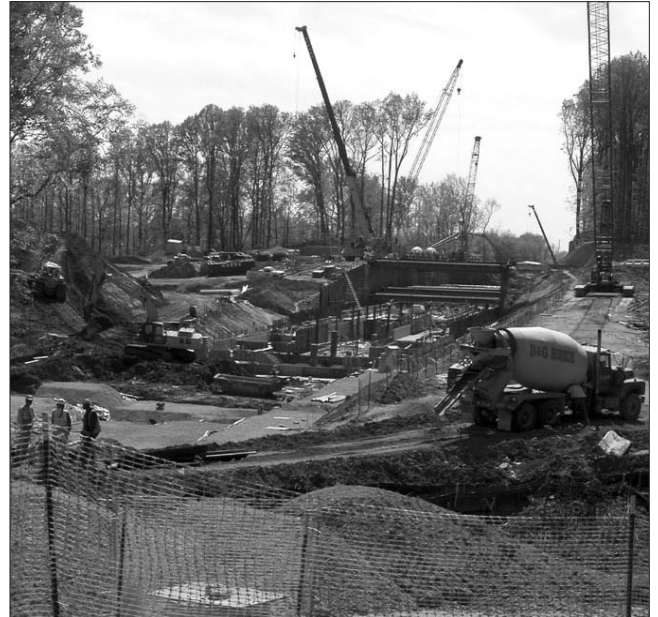
The Morgan Boulevard Metro Station under construction in early 2003.
