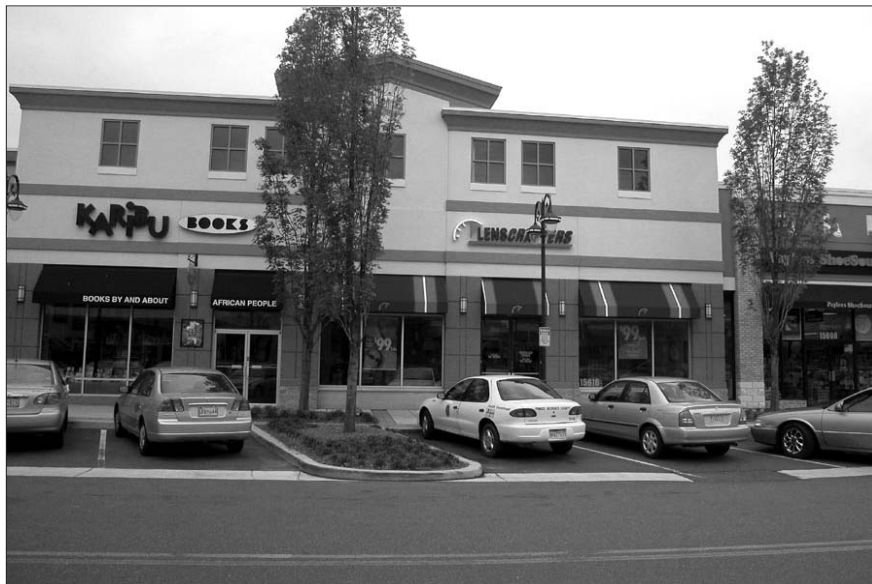
Curb bump-outs provide visual and physical separations from long lines of parked cars.
