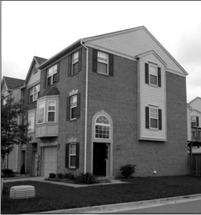
Endwall treatments such as projections, windows, and doors create visual interest and alleviate large, unfriendly expanses of walls facing public areas.
