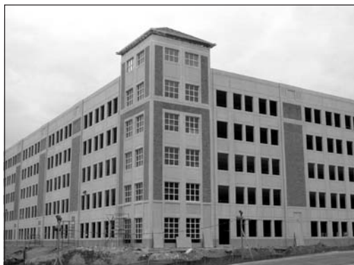
Garages designed to resemble traditional buildings are more pleasing than those designed with long, horizontal slot openings.
