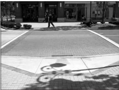
Crosswalks that continue sidewalk materials across streets make them more visible to motorists and further enhance pedestrian safety.
