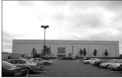
Monolithic, box-like structures such as this one should be avoided.
